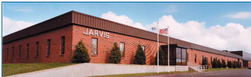
Jarvis' World Headquarters Building in Middletown, CT U.S.A.
