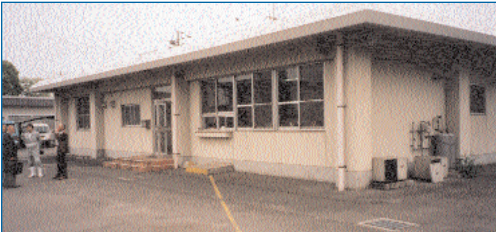
Fukuyama Municipal Abattoir's main office building. Fukuyama Municipal Abattoir is a leading Japanese meat processing company and a long-time Jarvis customer.
